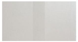
This term is used to describe the effect of the paint finish reacting differently on the joints to the surface of the board (suction), if the sealer is not applied the joints may be visible no matter how well the taping and jointing process has been completed. Once dry, a paint finish can be applied in the normal manner.
