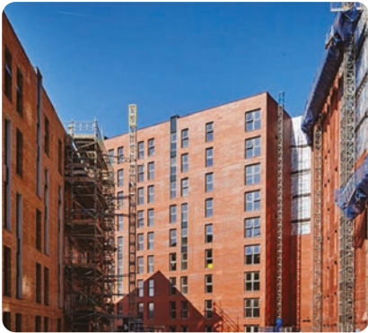
Brick cladding: University of Salford
