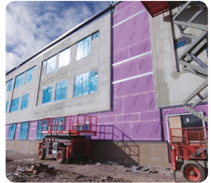
Insulated render: North Somerset Enterprise and Technology College
