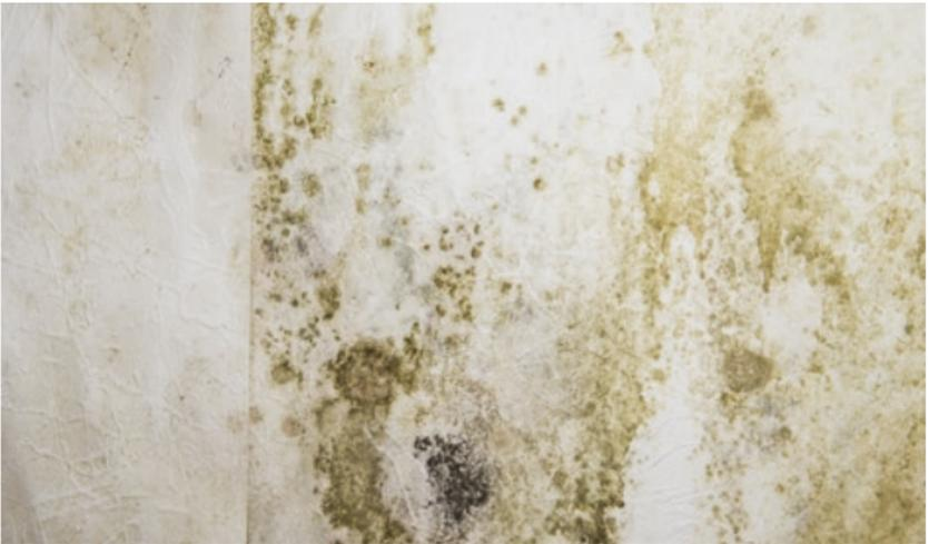
Typical example of mould growth on wall using incorrect plasterboard.
